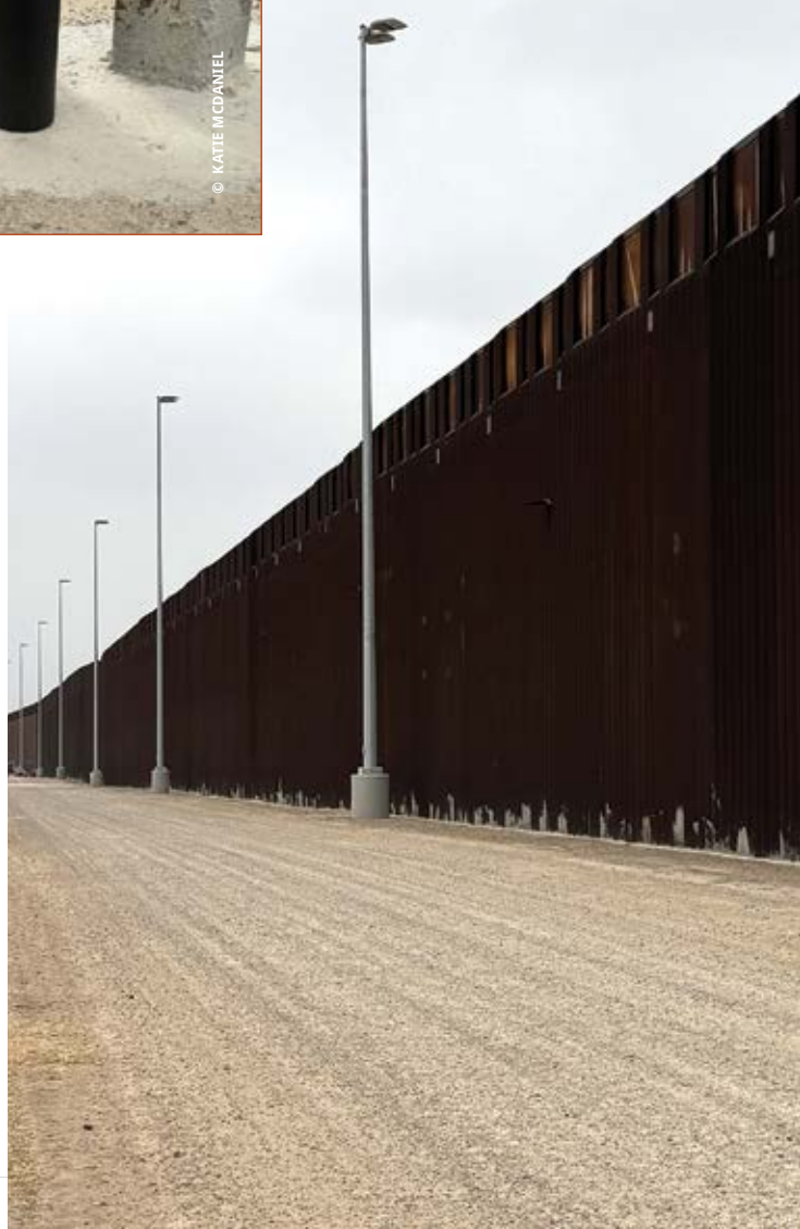
The border barrier system is a 30-ft tall metal structure equipped with lights, cameras, and vehicle patrols.
