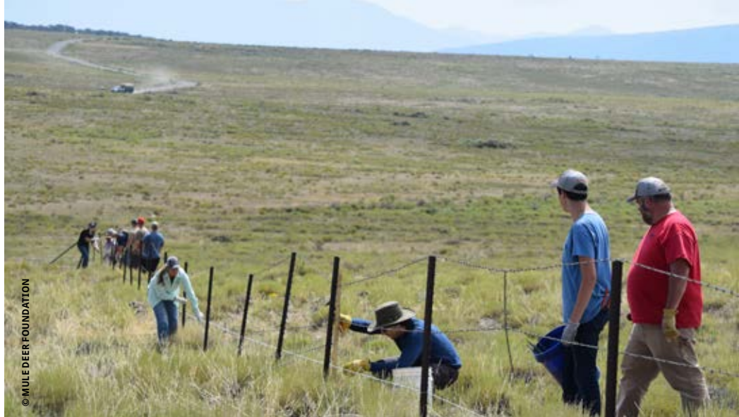
Pictured here, volunteers rebuild fences to wildlife-friendly standards. Fencing can be a barrier to movement, impede migrations, and cause injury or death to deer and other big game. Retrofitting fences is an extremely beneficial activity, particularly in migration corridors.
